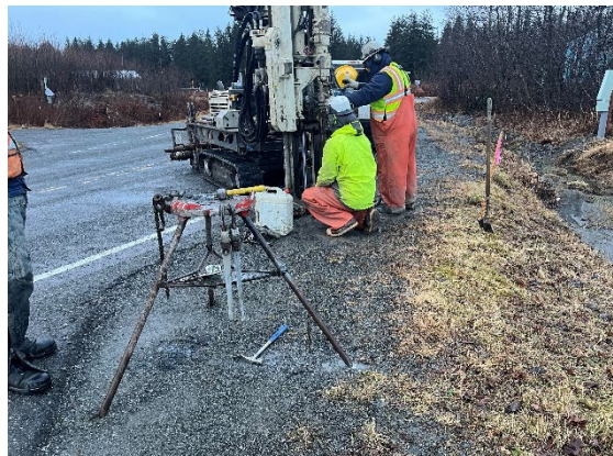
Exhibit 1: Setting up drill rig on the roadside.
