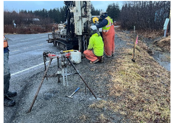
Exhibit 1: Setting up drill rig on the roadside.
