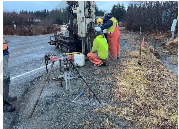
Exhibit 1: Setting up drill rig on the roadside.
